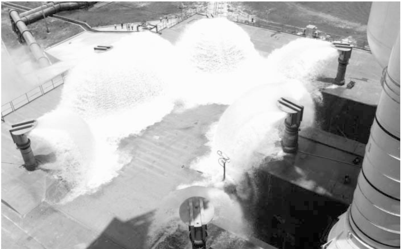
The rainbirds begin to place a cushion of water on the Mobile Launcher Platform to prevent reflection of acoustical energy from the Platform's steel structure. Fresh water stored in an elevated tank flows through a valve network (upper left) to achieve the proper pressure. It flows through the giant pipes to the rainbirds.
