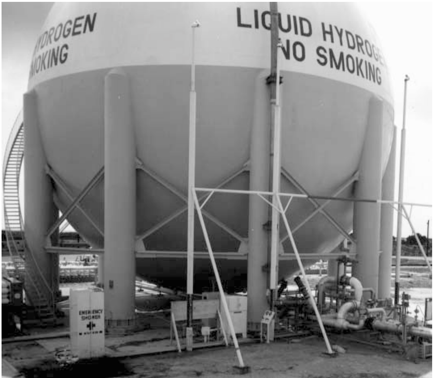
A large round container which is actually a high vacuum bottle stores the supercold liquid hydrogen at the launch pad. A similar round vessel holds the liquid oxygen. The liquid propellants flow to the orbiter's main engines.
