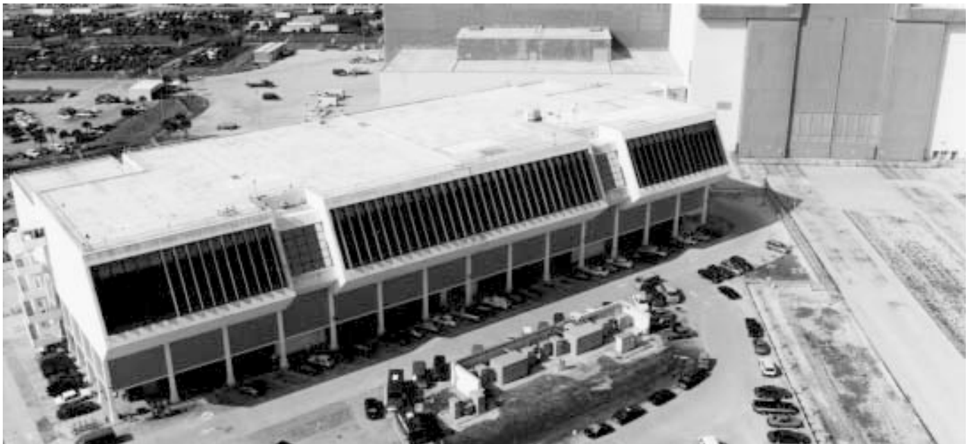
The Launch Control Center faces both launch pads.
