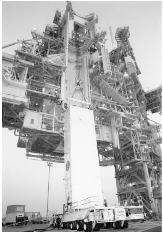
The Payload Canister is lifted from its Transporter into the Rotating Service Structure at the launch pad.
