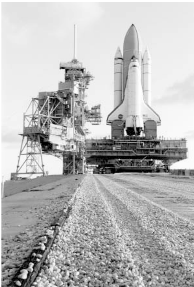
Space Shuttle Discovery atop its Mobile Launcher Platform waits on Launch Pad 39A for liftoff on mission STS-92. At left is the Rotating Service Structure in its open position.
