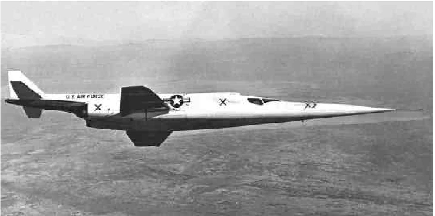
NASA Photo E-17348. In flight photo of the X-3, which made significant contributions to knowledge about inertial coupling.
