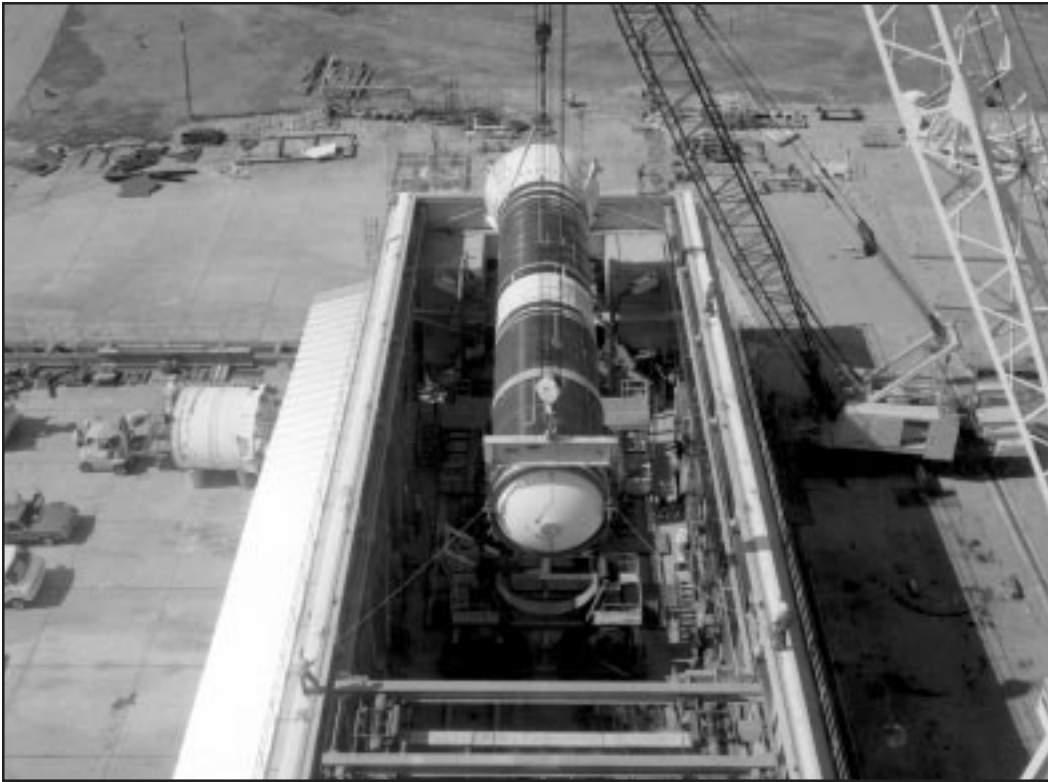
Lowering solid rocket booster into Marshall structural test stand.
